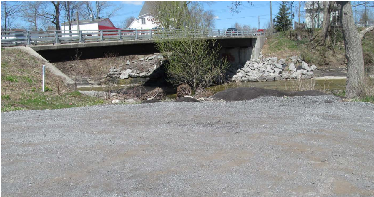
Parking lot (151 Borden Road).
